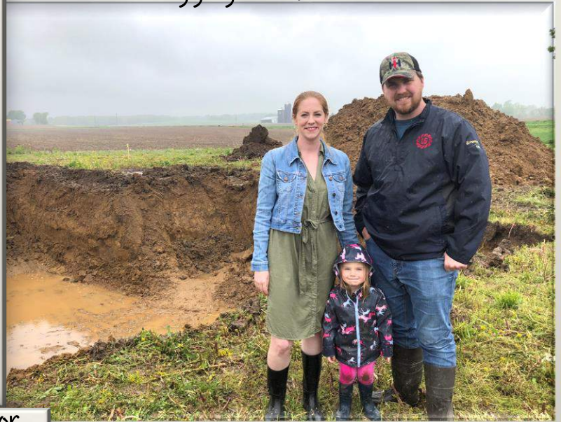
Digging Our Basement
